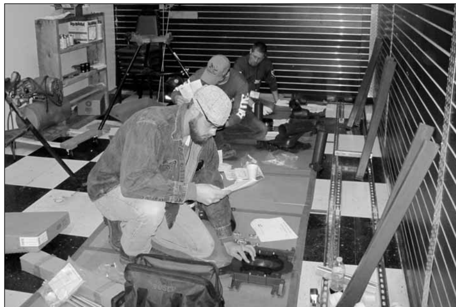
Plumber contestants set commercial toilet carriers during the WV State Pipe Trades Apprenticeship Contest held in Huntington. Pictured front to back: Jacob Dierkes, LU 152 Morgantown; Kyle Phillips, LU 565 Parkersburg; and Joe Battistelli, LU 83 Wheeling.
